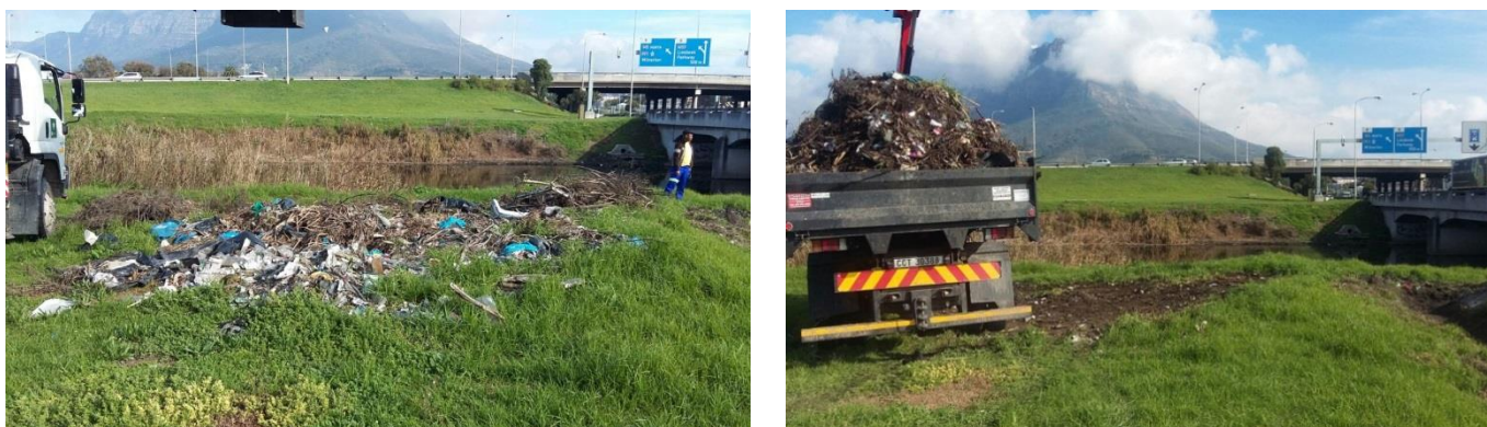
Figure 56: Cleaning rubble at Raapenberg bridge with new grab truck
