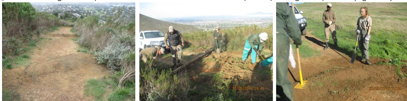
Figure 29: Construction of water bars as part of footpaths and road network maintenance
