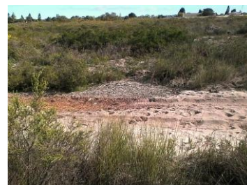
Figure 28: Recovering erosion site
