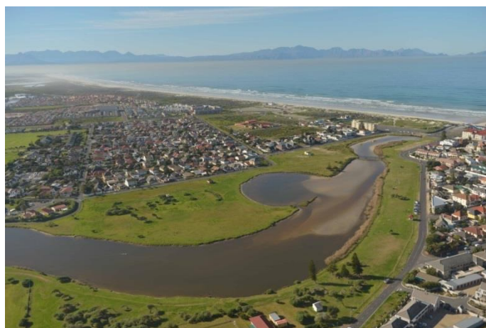
Figure 27: Zandvlei estuary showing siltation
