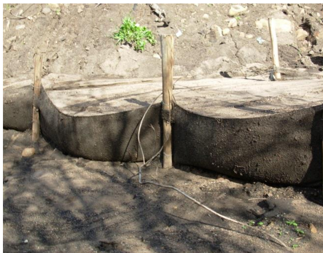
Figure 10: Silt curtain traps to prevent erosion installed by EPWP team
