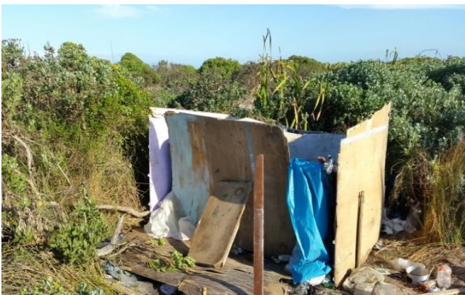
Figure 8: Illegal structure in Zandwolf section of the False Bay Nature Reserve
