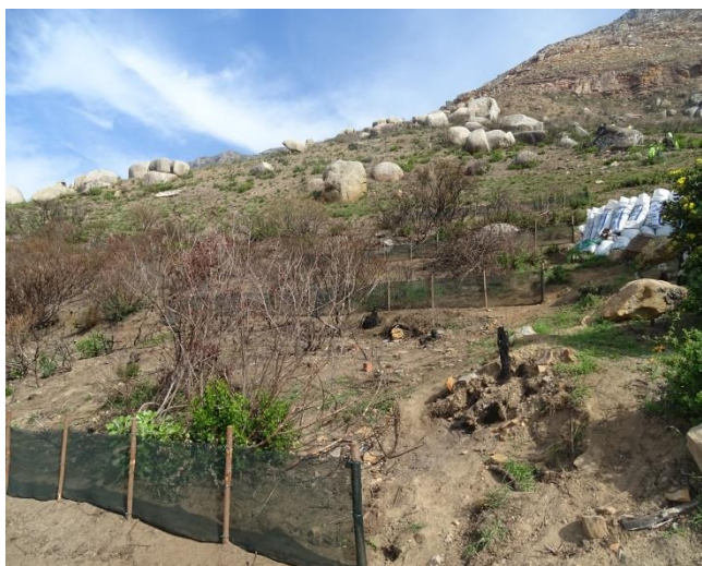
Figure 9: Installation of silt curtains in Simon's Town by EPWP workers
